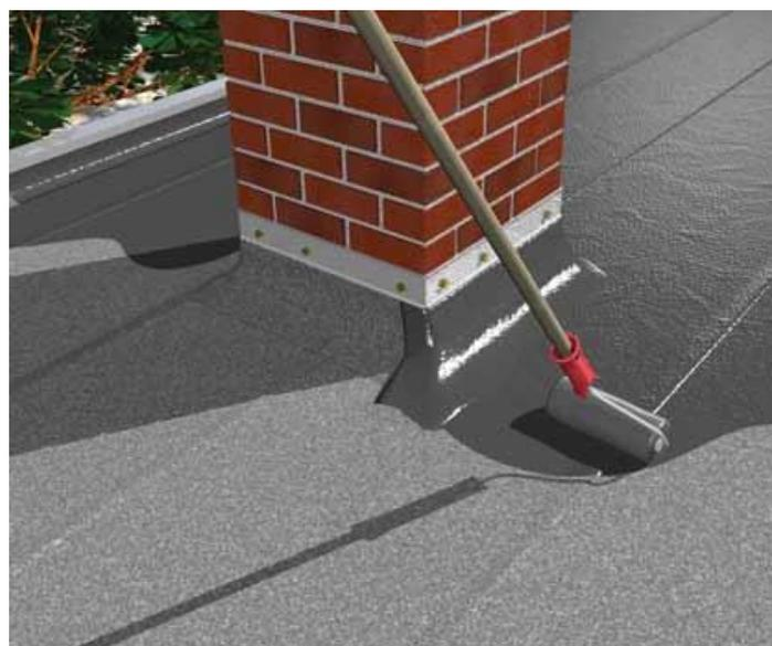
Figure 1. Epoxy based waterproofing application
